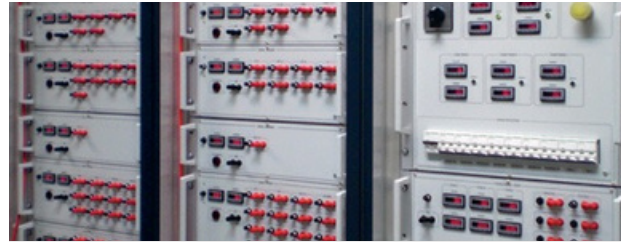
Support Center for NH90 Power racks to control the distribution of 115VAC/400Hz and 28VDC
