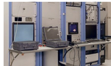
Integration rig for maritime patrol mission LRU (Line Replacement Units) racks
